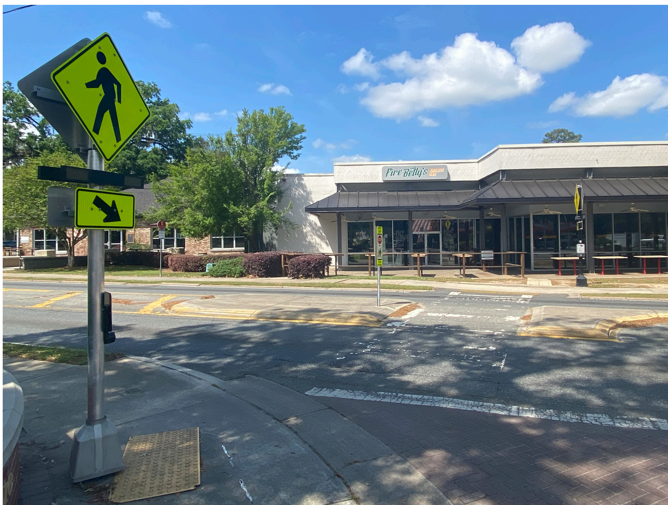
Rectangular Rapid Flashing Beacon (RRFB)
