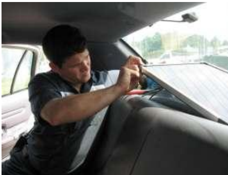
A City of Kingsland mechanic installs a solar panel on the rear deck of a patrol car.
