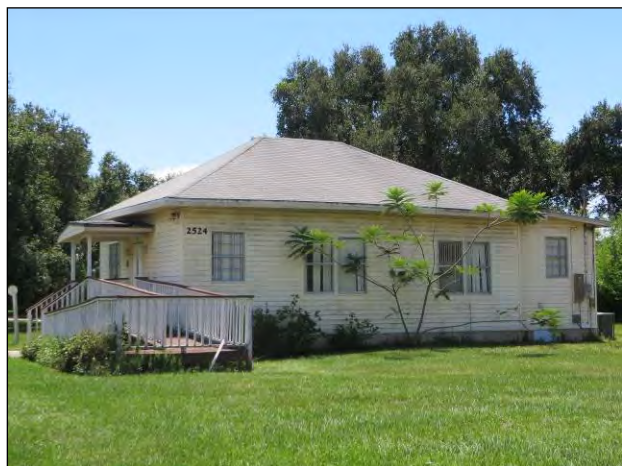
Figure 28. Resource 8OS02971 provides an example of the Frame Vernacular style within the Neptune Road APE. Photograph facing west.
