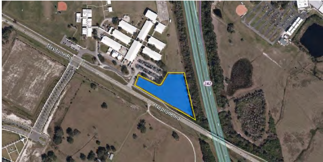
Photo 6: Aerial photograph of pond location 2C located 300 ft NW of the Neptune Overpass of Florida's Turnpike on the Neptune Middle School Campus.
