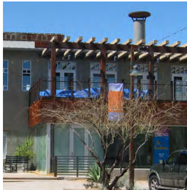
Steel, wood and wire mesh balconies
