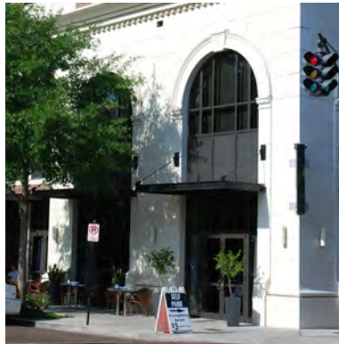
Two-story office building
