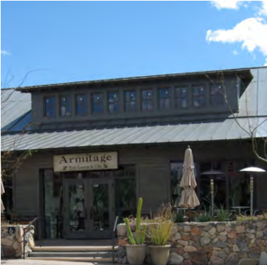
Shed-style dormer windows
