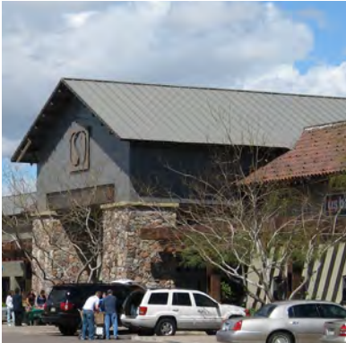
Rooflines similar to barns + agricultural buildings
