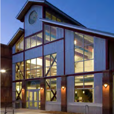
Clerestory with barn-shaped rooflines
