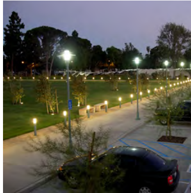
Pedestrian overhead + bollard lighting
