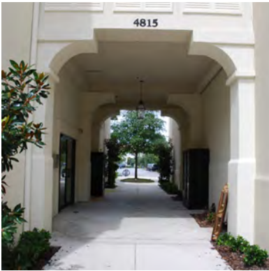
Pedestrian covered walkway
