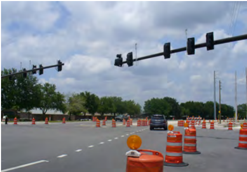
Narcoossee Road construction
