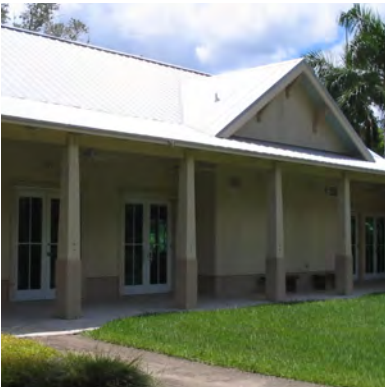
Deep building overhangs
