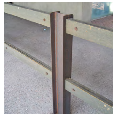
Steel beam posts + wooden rails
