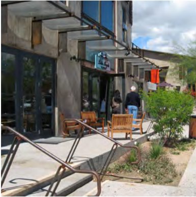
Steel + glass awnings
