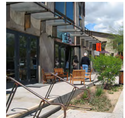
Steel + glass awnings
