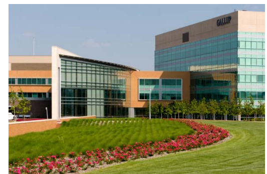
High Tech Office Campus
